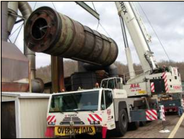
New Furnace Installation at Wood Pellet Plant
