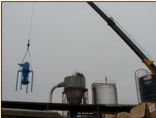
Sawdust Storage Bin Assembly and Installation
