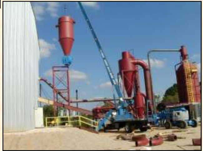
Installing Refurbished Drum Dryer For Sawdust
