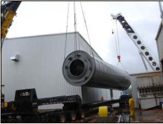
Cyclone Field Assembly and Installation by Energy Unlimited Inc
