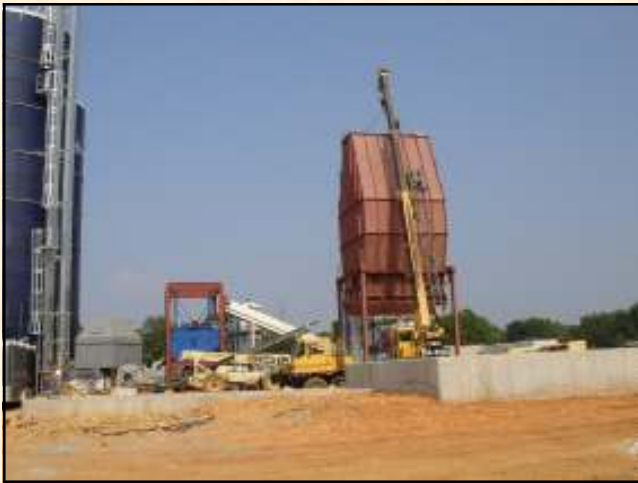
Sawdust Storage Bin Installed By Energy Unlimited Inc
