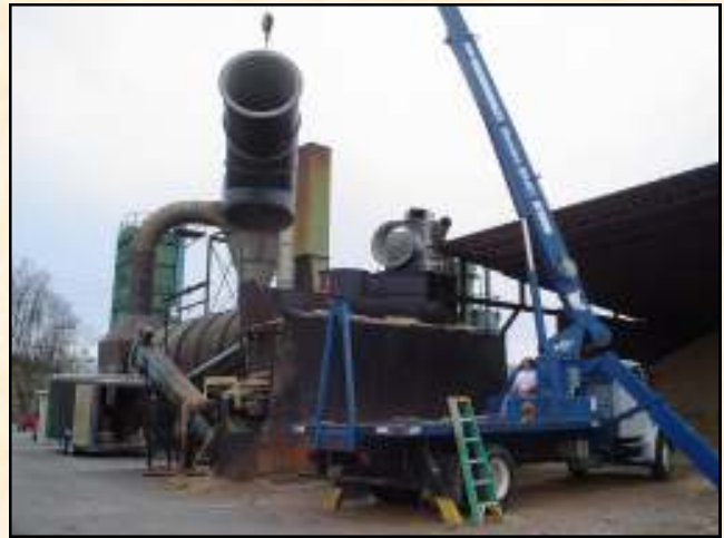
Replacing worn out Dryer With New Rotary Dryer
